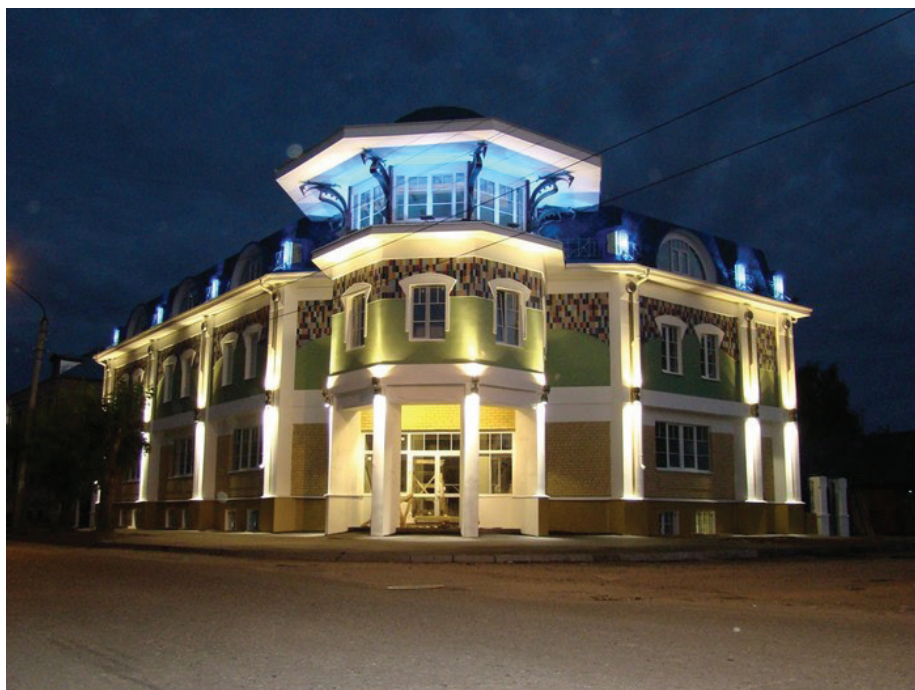
Pic. 2. Local lighting of the building [5].
