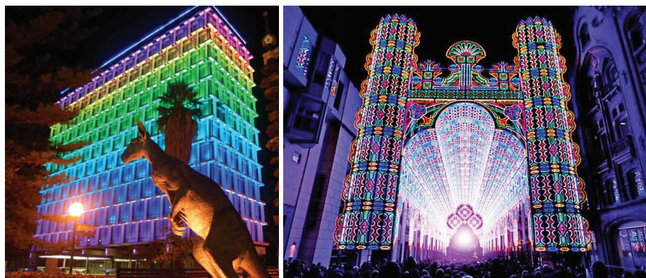
Fig. 3. Hidden lighting of the building [5]. Plant elements lighting.
